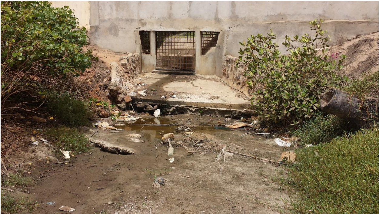
Figure 14: The Discharge Point of the Senegambia Storm Drain
