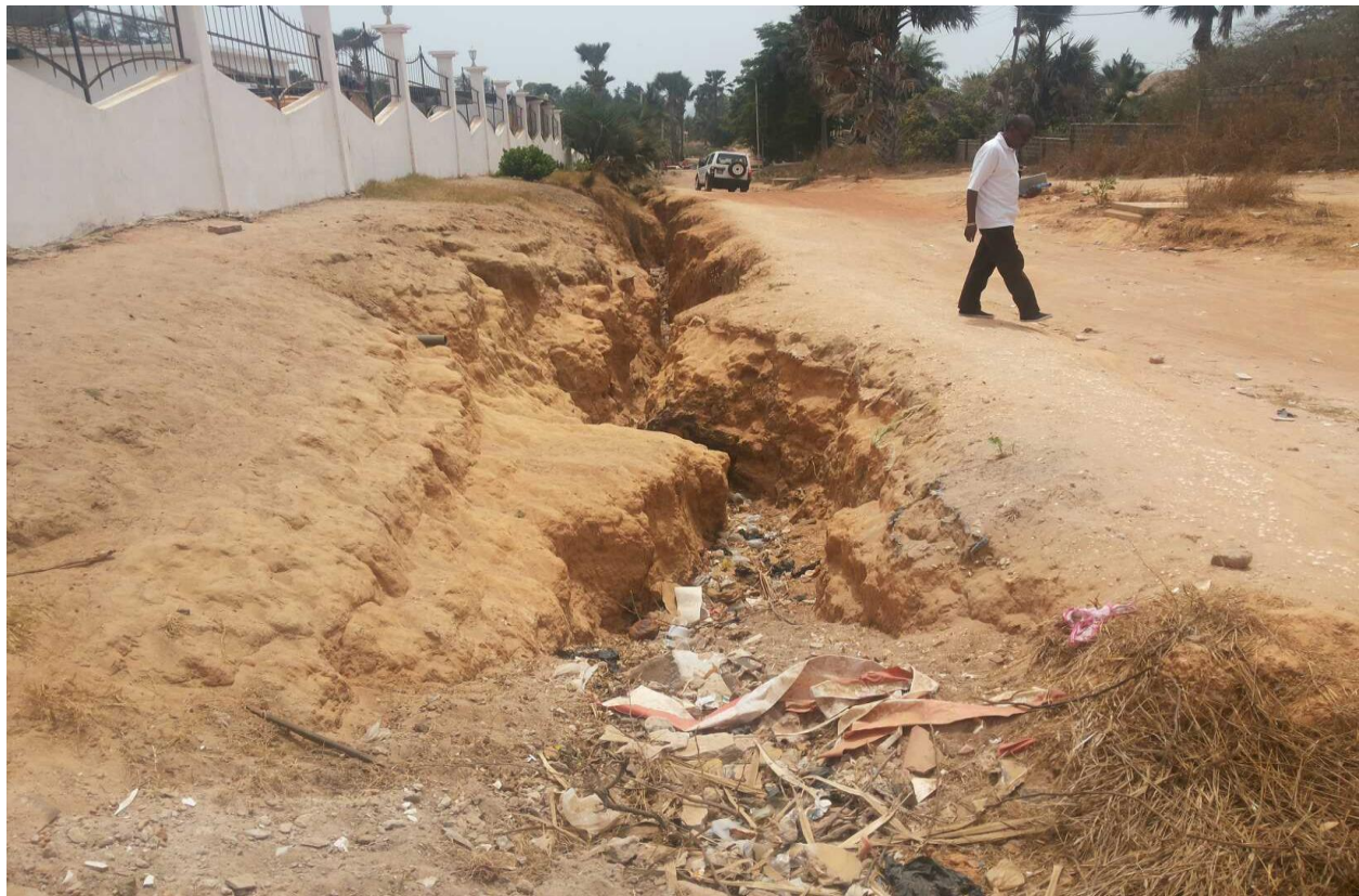
Figure 12: Photo of gully by the fence of Galaxy Entertainment Park created by storm water arising from the highway and Kololi
